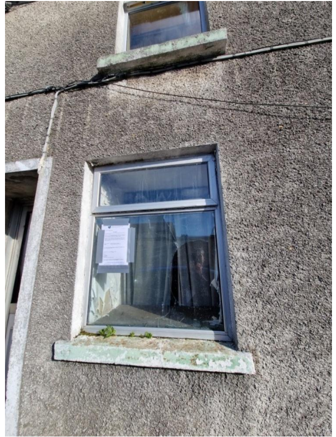
Images E & F above from 24 th February 2025, Section 8(2) posting onsite, facia & window sills stained / dirty & window broken.
