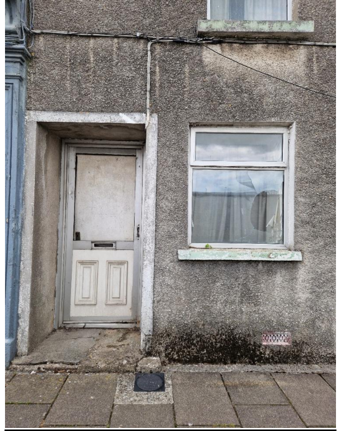
Images A & B above 30 th July 2024: Front views of the property from Church St., Cappoquin, showing, damaged shuttered up doorway, letterbox and ironmongery missing, ground floor window broken and façade stained and dirty.
