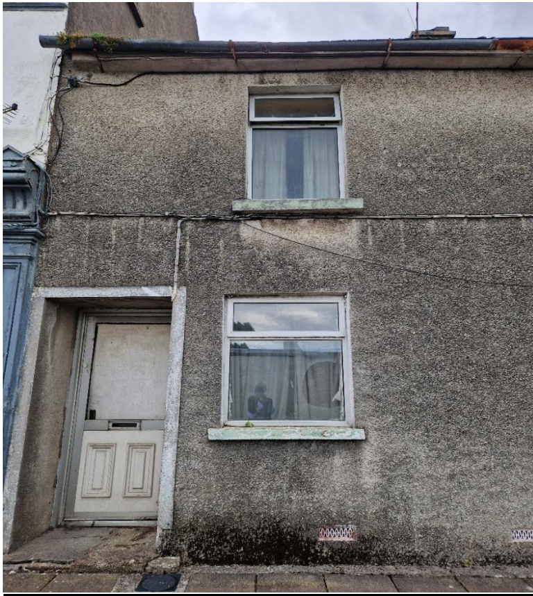
Images A & B above 30 th July 2024: Front views of the property from Church St., Cappoquin, showing, damaged shuttered up doorway, letterbox and ironmongery missing, ground floor window broken and façade stained and dirty.
