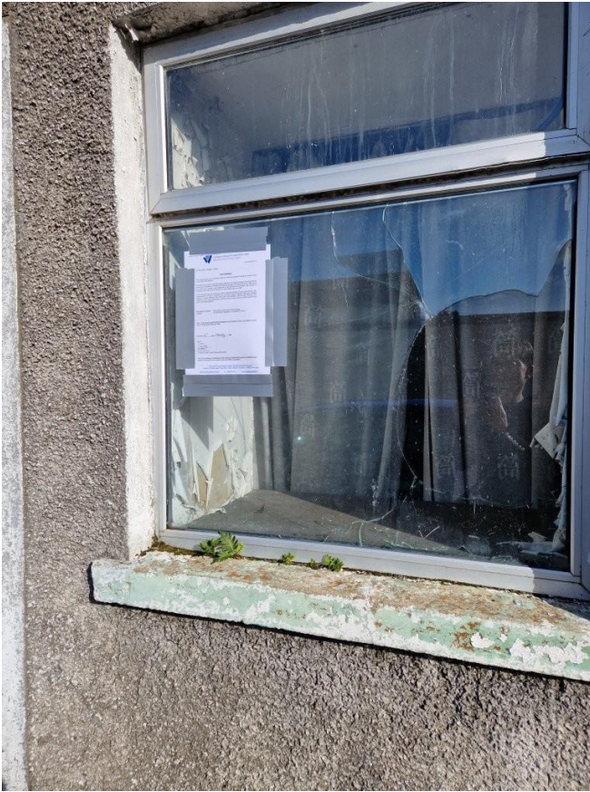
Images E & F above from 24 th February 2025, Section 8(2) posting onsite, facia & window sills stained / dirty & window broken.
